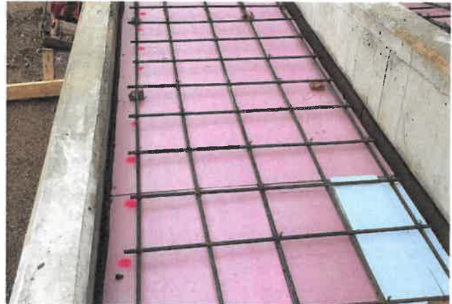
Birnamwood Elem Ramp Concrete
