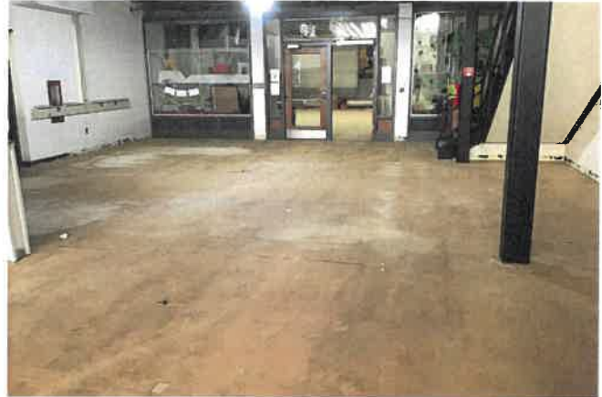
HS Flooring Demolition At The Library
