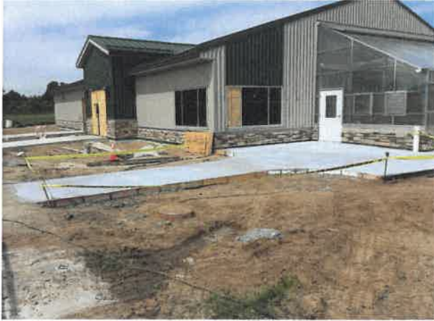
Ag Building Concrete Work and Stone Veneer
