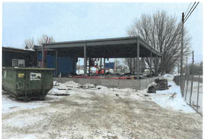
Birnamwood Elem Structural Steel
