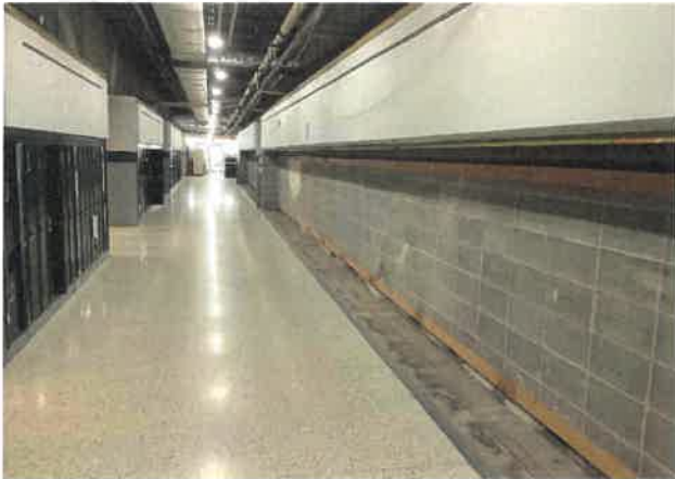
Interior High School Work
