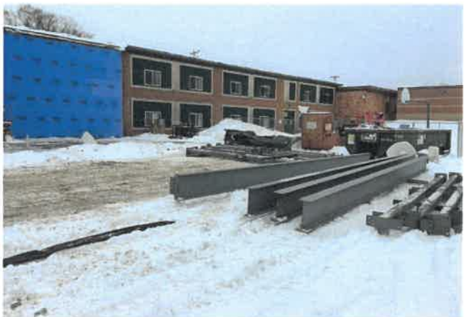
Wittenberg Elem Structural Steel
