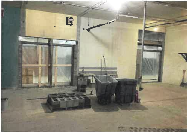
Interior High School Work
