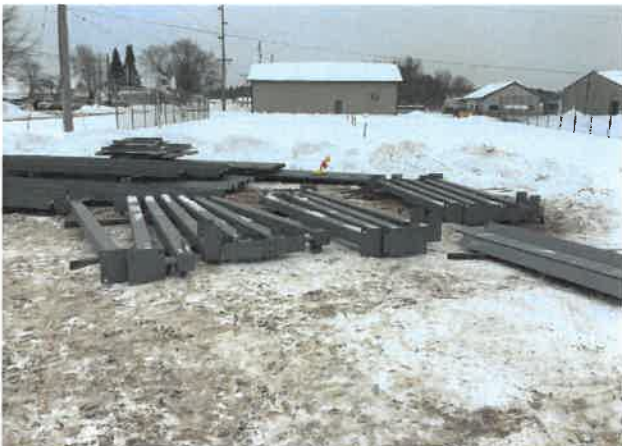
Birnamwood Elem Structural Steel
