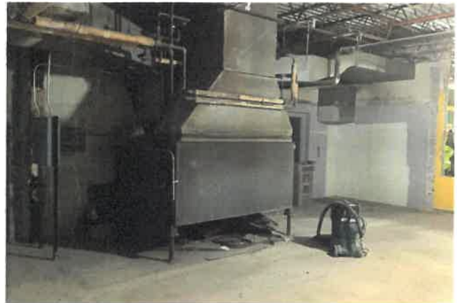
High School Mechanical Demolition
