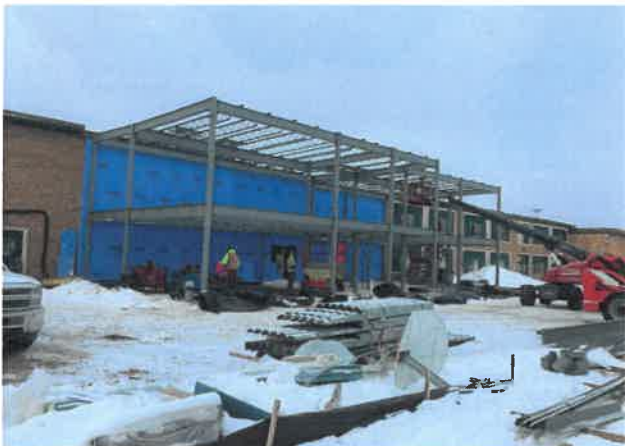
Wittenberg Elem Structural Steel
