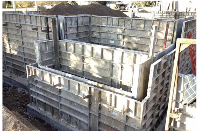
Forming and wall prep for a Friday wall pour
