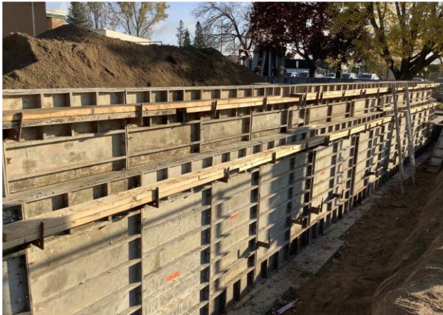
Wall forming at Birnamwood Addition
