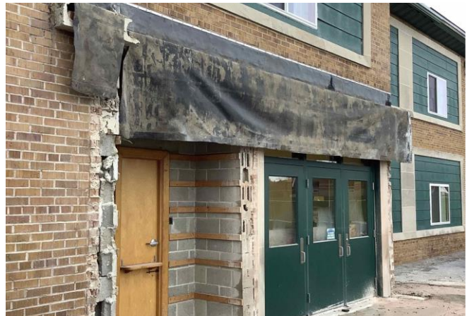
Demo to make ready for foundations
