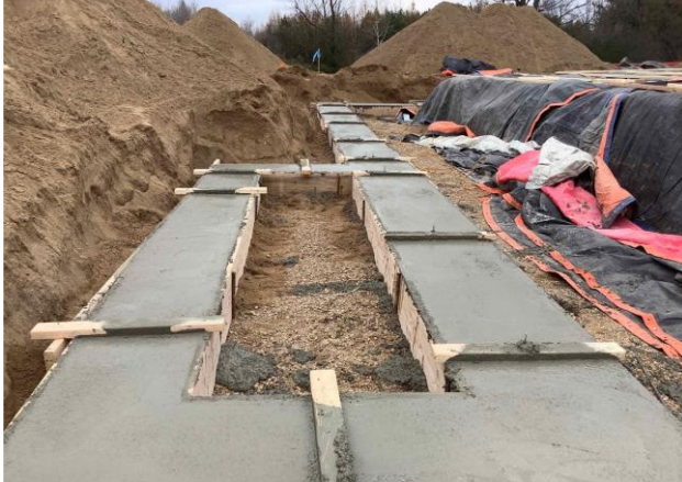
Enviro building north wall footings
