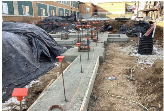
Witt Elem addition footings
