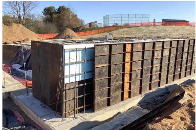
Enviro building foundation walls
