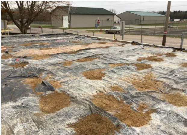
Birnamwood backfilled and covered
