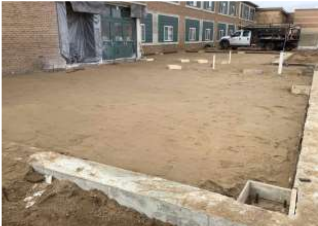
Witt Elem concrete floor prep
