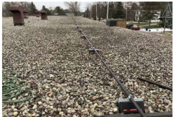
Mechanical gas piping on going at all sites
