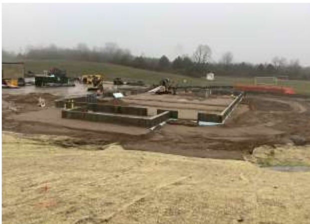
Witt HS grading and underground plumbing
