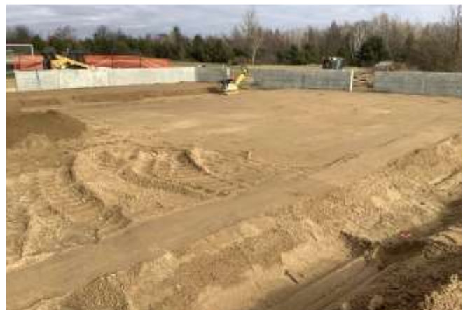
Enviro building backfill and floor prep
