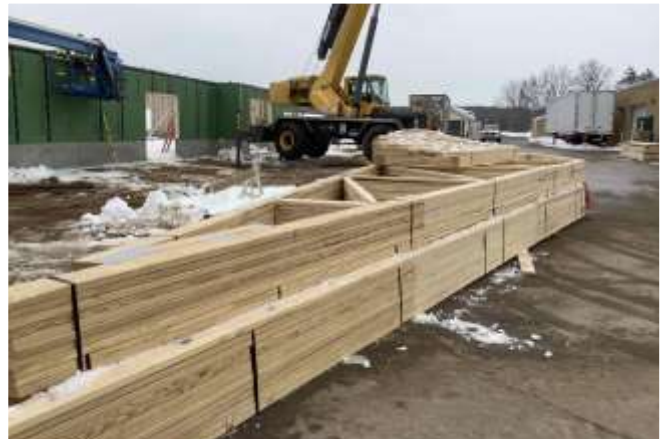
Enviro building roof trusses
