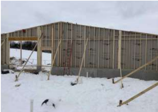
Enviro Building wall framing
