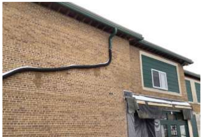
Witt Elem Roof demo
