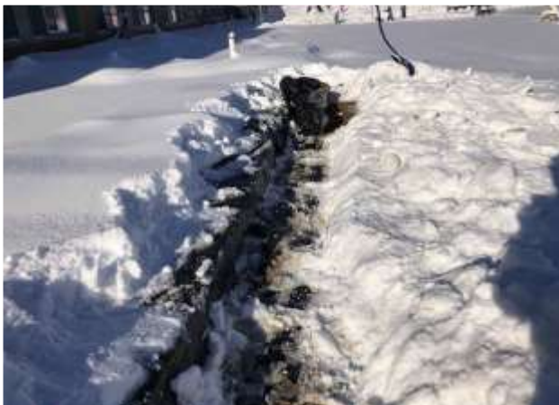
Witt Elem shoveling out
