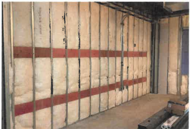
Birnamwood Elem interior ready for drywall
