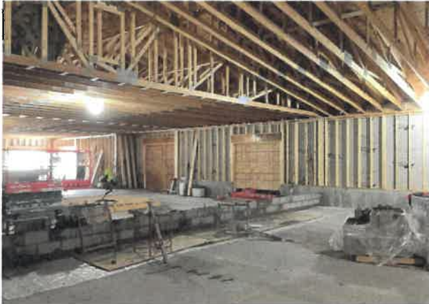
High School Enviro Building
