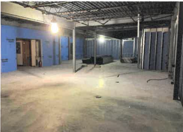
Wittenberg Elem upper floor ready for framing
