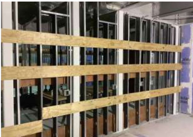
Wittenberg Elem ready for drywall
