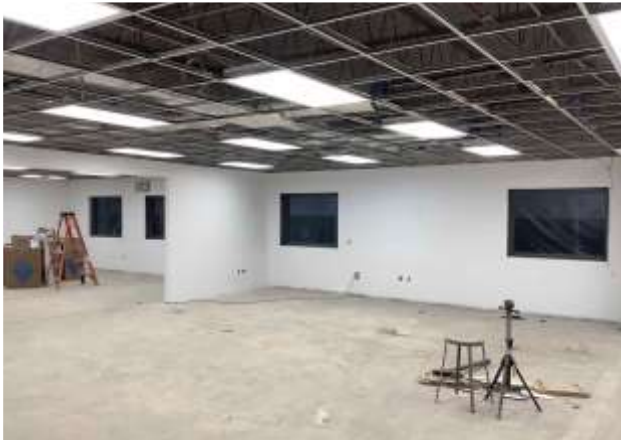
High School classrooms
