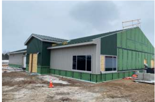
High School Ag Building
