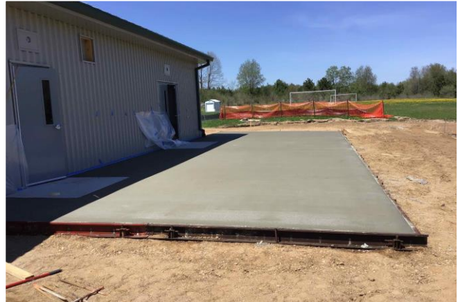
Ag Building Exterior Concrete
