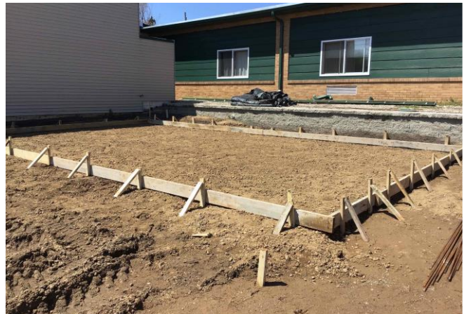
Birnamwood Elem Grading & Exterior Concrete
