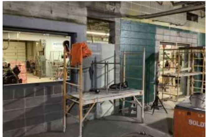
High School Masonry
