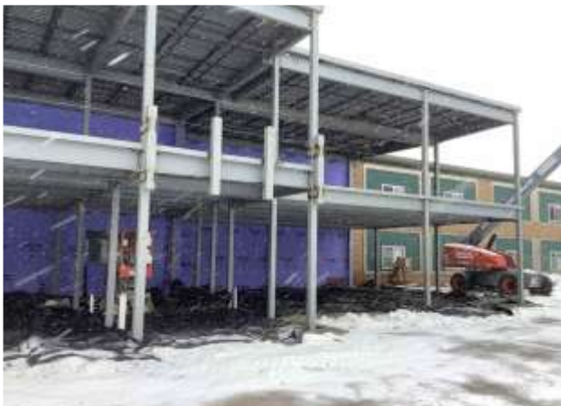
Wittenberg Elem Structural Steel Complete
