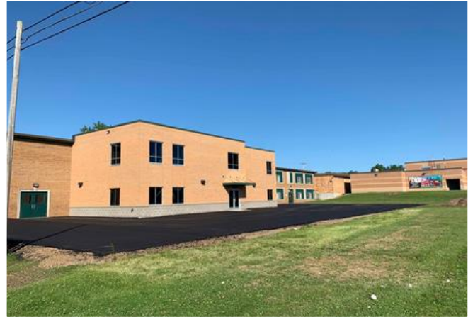
Wittenberg Elementary Addition
