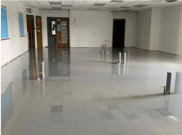
HS Epoxy Floors (Science Rooms)
