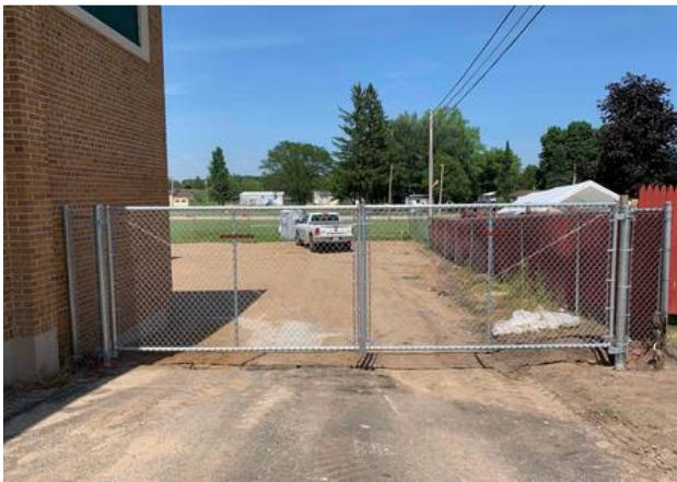
Witt Elementary New Gate
